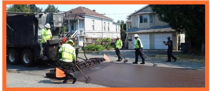
Example: microsurfacing pavement repair work.
